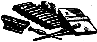
FIG. 9.—Currying Apparatus. C, pommel; R, raising board; S, slicker.
